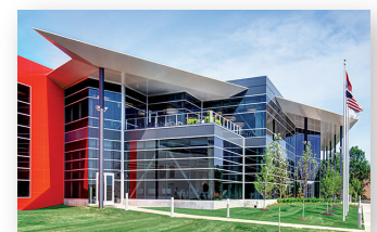
2016 Watlow's headquarters and Advanced Technology Center following a complete renovation
